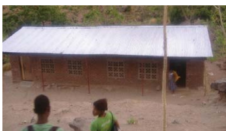
Newly-roofed school in Thoto Msinge thanks to Palmer and Howells
